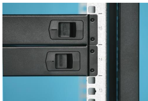
Visible U marks after installation.
